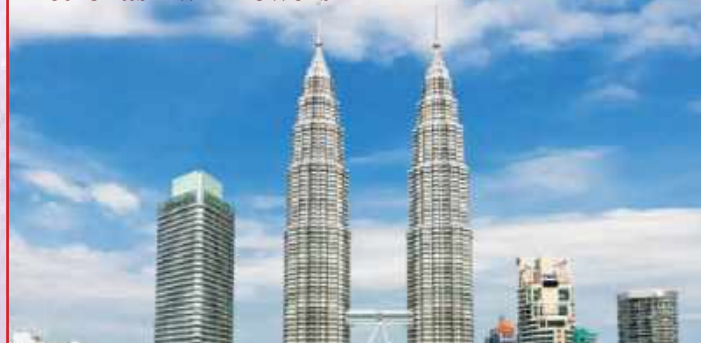
Petronas Twin Towers
