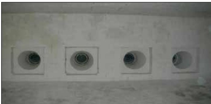
Refractory lining and burner blocks after coating with ESPON-RCP
